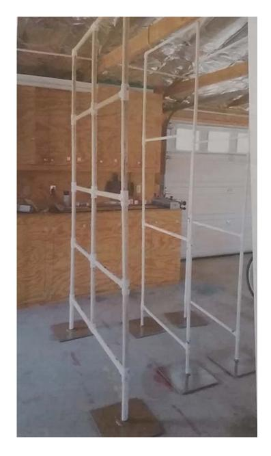
If you have room on stage for your PVC frames to have feet that stick out farther than 6 inches from center as they do when using the steel plate bases, OR if you want to be able to flip the pieces around and / or have them be light enough for a youth to pick up and move easily, you can use feet instead of bases. We did for most productions. Parts for these frames are shown in this and the next page.
